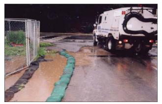
As you guessed, there was a storm which exceeded the capacities of the project BMPs (Best Management Practices). The retention basin constructed to catch storm water overflowed and cloudy water reached a nearby drain inlet. The contractor properly contacted its SWPPP consultant, who recommended draining the basin manually using a filter bag over the end of the drain outlet. That was done, but a governmental inspector "happened" by and noticed the cloudy discharge.
